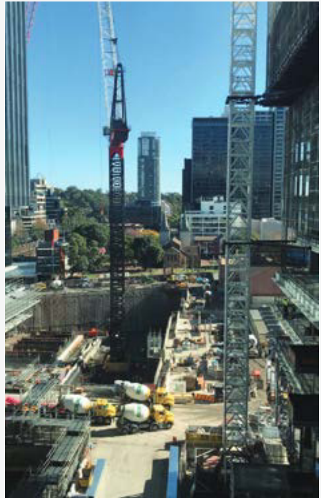
View of construction activity at Parramatta Square in 2019
